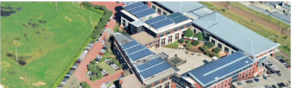
Grid-tied PV system at Black River Park.
